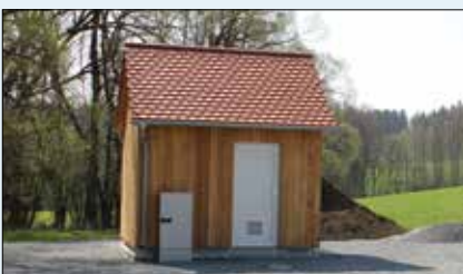
Example: Installation in a Machine house
